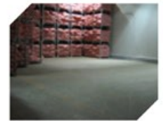
CPAC Freezing Room Concrete
