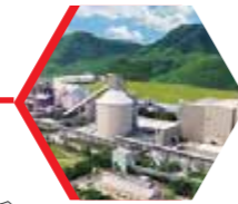
SÔNG GIANH Integrated Plant
